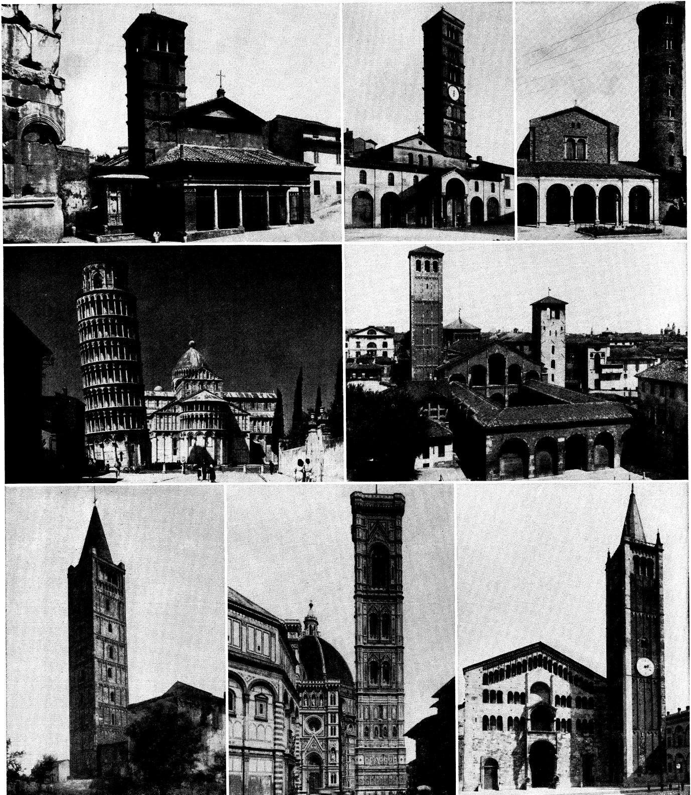
PHOTOGRAPHS (ALL EXCEPT CENTRE LEFT AND BOTTOM CENTRE) AL NARI, (CENTRE LEFT) G. E. KIDDER SMITH. (BOTTOM CENTRE) EWING GALLOWAY
