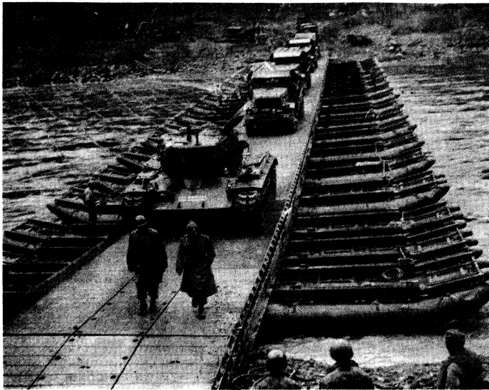
U S ARMY PHOTOGRAPH BY COURTESY OF THE CORPS OF ENGINEERS FIG. 3.— MEDIUM TANK AND BRIDGE TRUCKS CROSSING A CLASS 60 FLOATING BRIDGE
