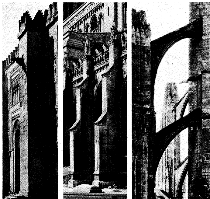
(LEFT) THREE LIONS, INC.; (CENTRE) A. F. KERSTING; (RIGHT) EWING GALLOWAY BUTTRESSES: (LEFT) ENGAGED COLUMN. GREAT MOSQUE, CORDOBA, SPAIN. 8TH CENTURY; (CENTRE) SLOPING BUTTRESSES. PETERBOROUGH CATHEDRAL. ENG.. 12TH CENTURY; (RIGHT) FLYING BUTTRESSES. CATHEDRAL OF ST. GATIENS. TOURS. FRANCE. 12TH–16TH CENTURIES
