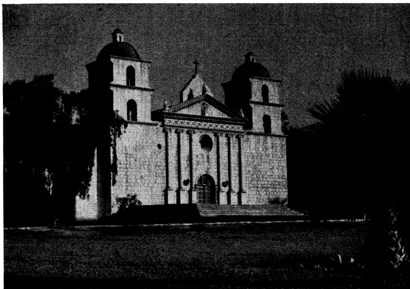
The mission at Santa Barbara, one of the most interesting examples of Spanish architecture in the state. Constructed of native sandstone, the mission was built in 1815
